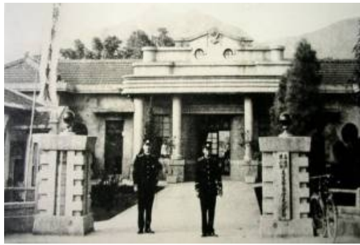
Fig. 10. Once mistakenly recognized as the only Japanese police station in Meinong was actually the third installation of the colonial law enforcement. Source: Meinong zhenzhi bianji weiyuan hui, Meinong zhenzhi (The Gazetteers of Meinong), (Meinong: Meinong zhengong suo, 1997), 1153.
